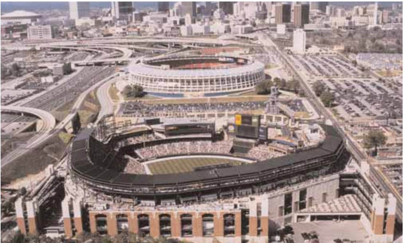
Fig. 13. In foreground, Atlanta Braves Baseball Stadium (formerly the Olympic Stadium), Atlanta Georgia (1996). Background left corner is the Georgia Dome which was also designed by CEG. Note that the old Atlanta-Fulton County Stadium (middle of picture above front stadium) has since been torn down.
