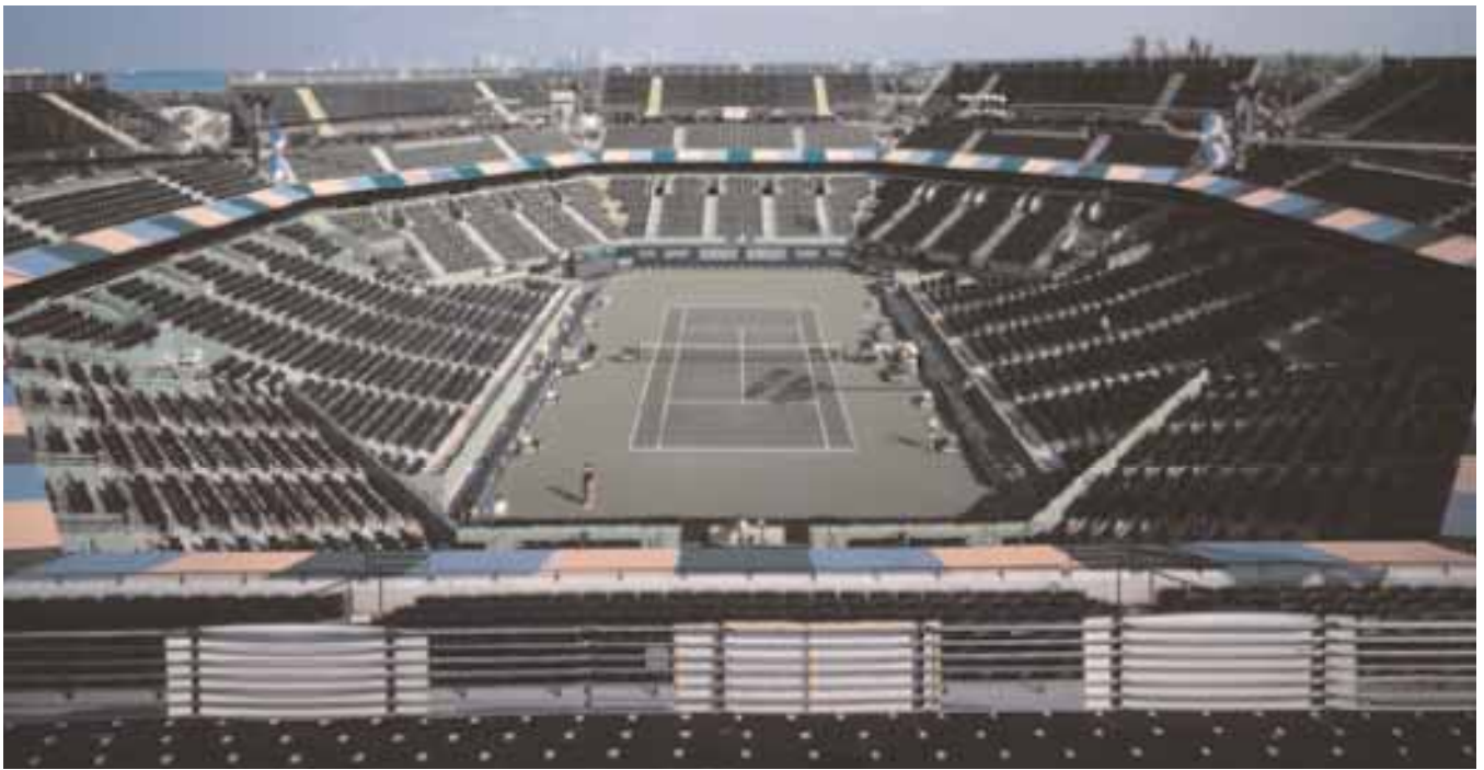
Fig. 11. Connecticut Tennis Center, New Haven, Connecticut (1991).
