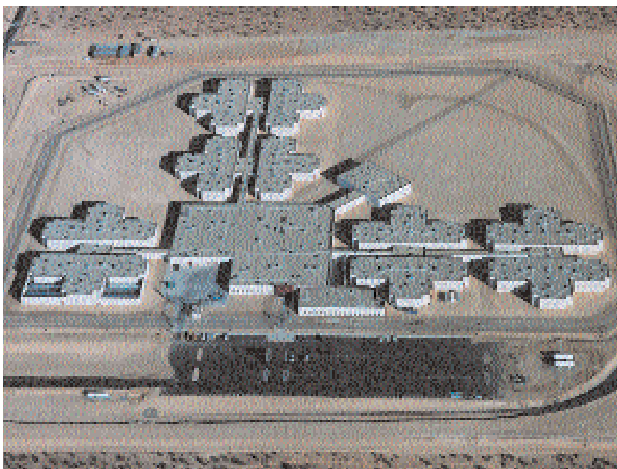
Fig. 16. CCA California Prison, California City, California (1997). This project was a CEG-Texas job.
