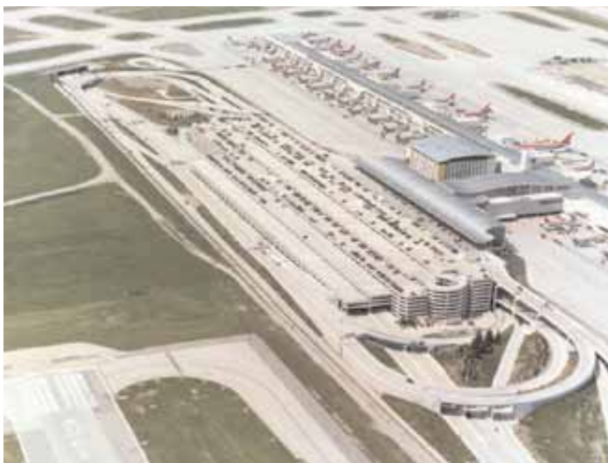
Fig. 15. Midfield Terminal parking structure (world's largest), Detroit, Michigan (2000). This project was a CEG-Texas job.
