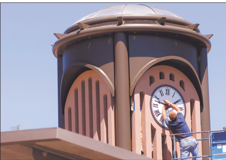
A worker makes adjustments to the clock tower on the new Vacaville Transit Plaza at East Monte Vista Avenue.
